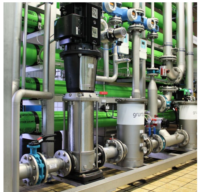
Pre-treatment for reverse osmosis in seawater desalination
