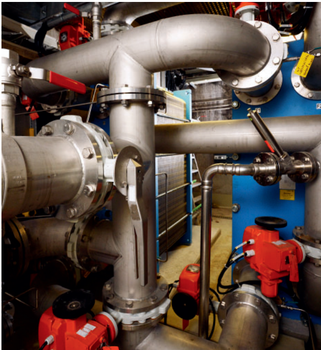
The vapour is fed into the local heat network via heat exchangers
