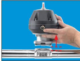
2. Loosen the valve body, diaphragm and / bonnet bolts diagonally and remove the actuator / bonnet from the valve body.
